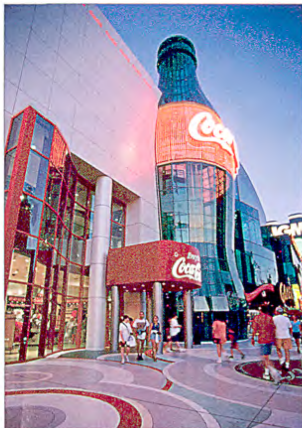
Creating a brand experience: Everything Coca-Cola in Las Vegas, with a 100-foot lighted Coke bottle as part of the front of the building.
